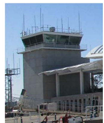
Airport Beacon atop the ATCT
