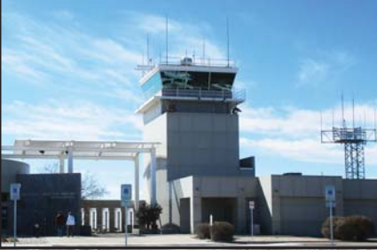
1 AIRPORT TRAFFIC CONTROL TOWER
